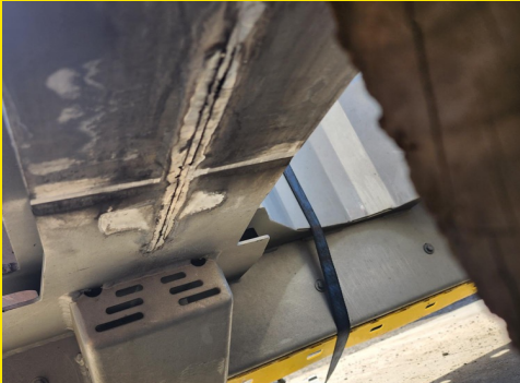
Cracked/damaged H-beam.
